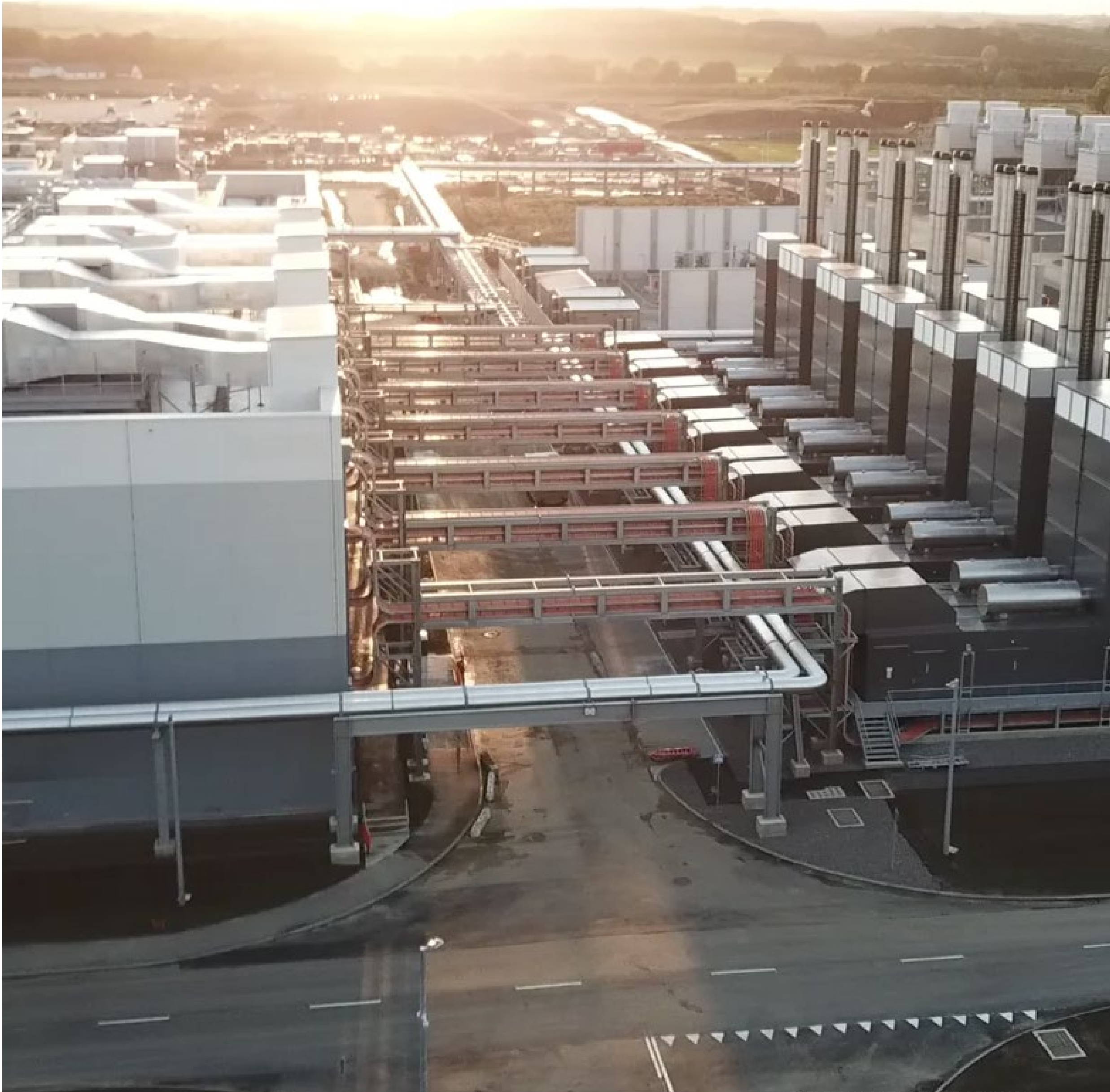
FREDERICIA DATA CENTRE, DENMARK
