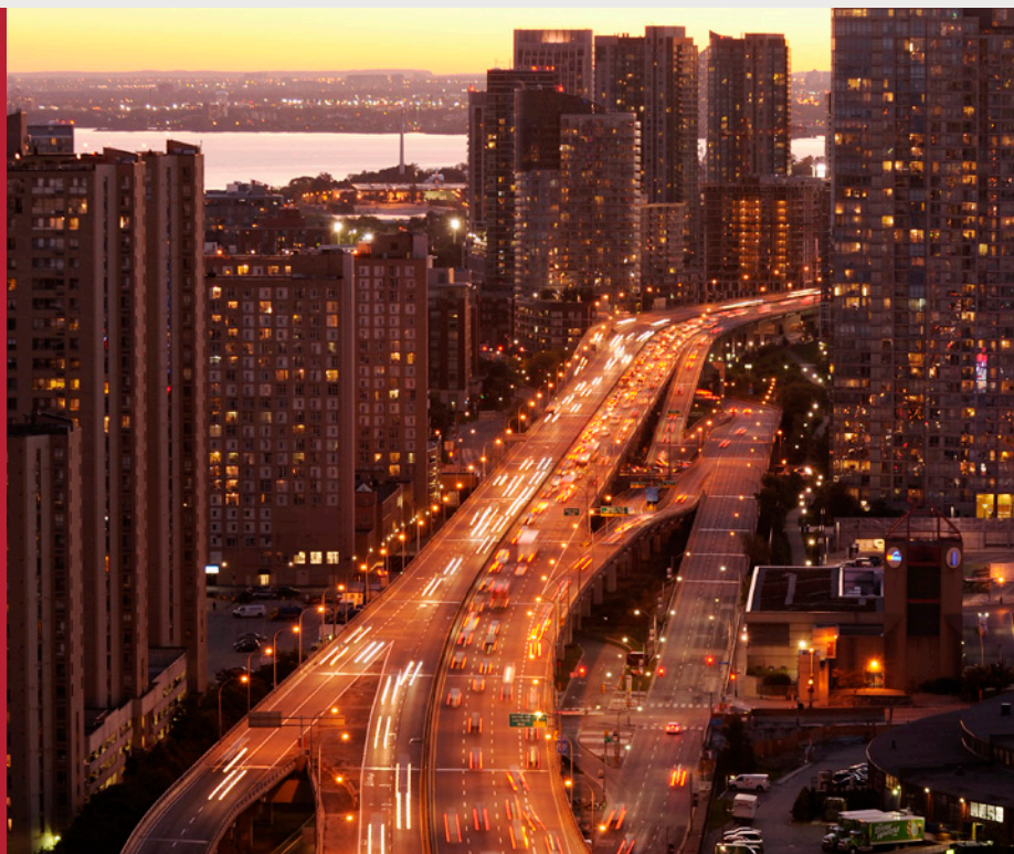
The Gardiner Expressway and downtown Toronto.
